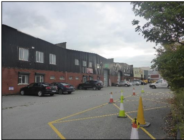
Plate 11.1 View of southern segment from Cookstown Estate Road
