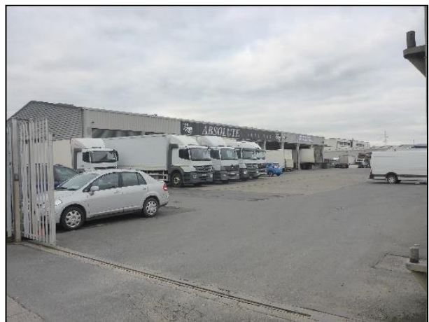
Plate 11.4 South corner of site
