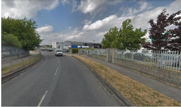
Plate 7. View North along Cookstown Road
